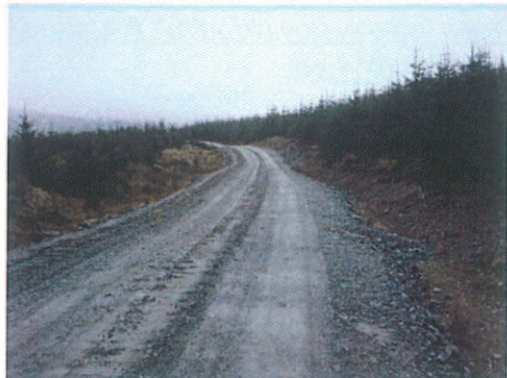
6. Looking North back along C262
