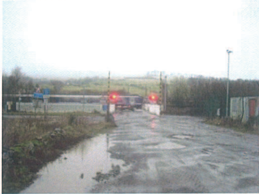
View of the level crossing on Moss Road showing working lights and barrier
