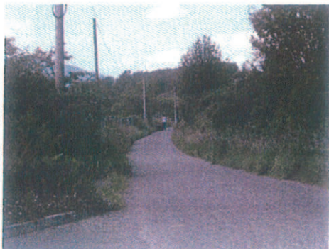
The road is currently used by pedestrians and cyclists
