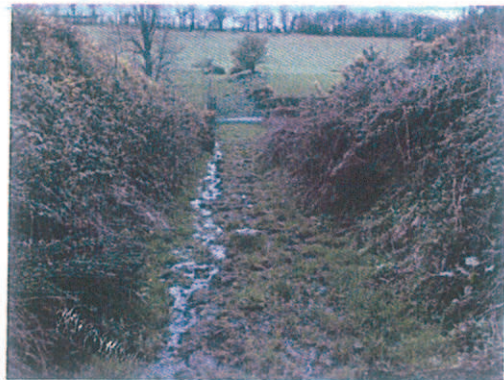
Path is poorly drained and steep
