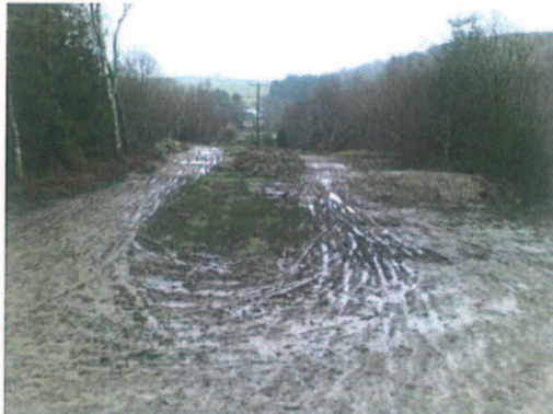
Open area under power cables appears to be used as a motorcycle track
