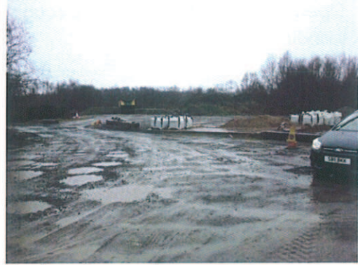
Engineering yard area
