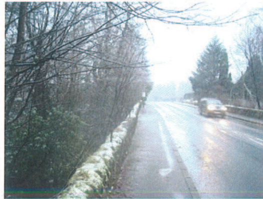
Typical narrower section of pavement cycle route marked by white line on road carriageway
