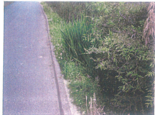
The road verge on Rosneath Rd can be very narrow in places and does not allow pedestrians to stand clear of cars
