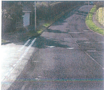
1. East Lennox Drive junction
